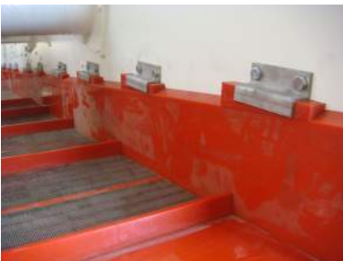
Side liners wedges and panels
